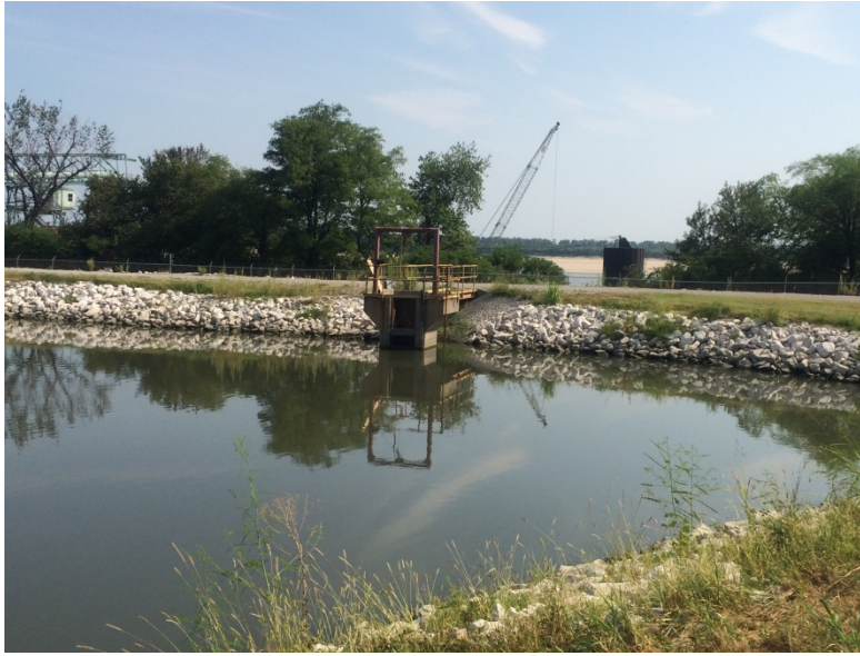
Photograph No. 11 Pond 004 Concrete drop inlet spillway with stoplogs Mississippi River in background
