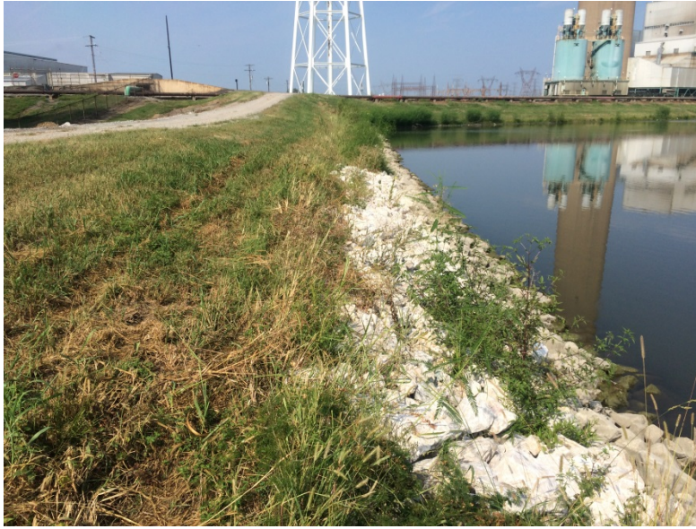
Photograph No. 9 Pond 004 Upstream slope with riprap and vegetation
