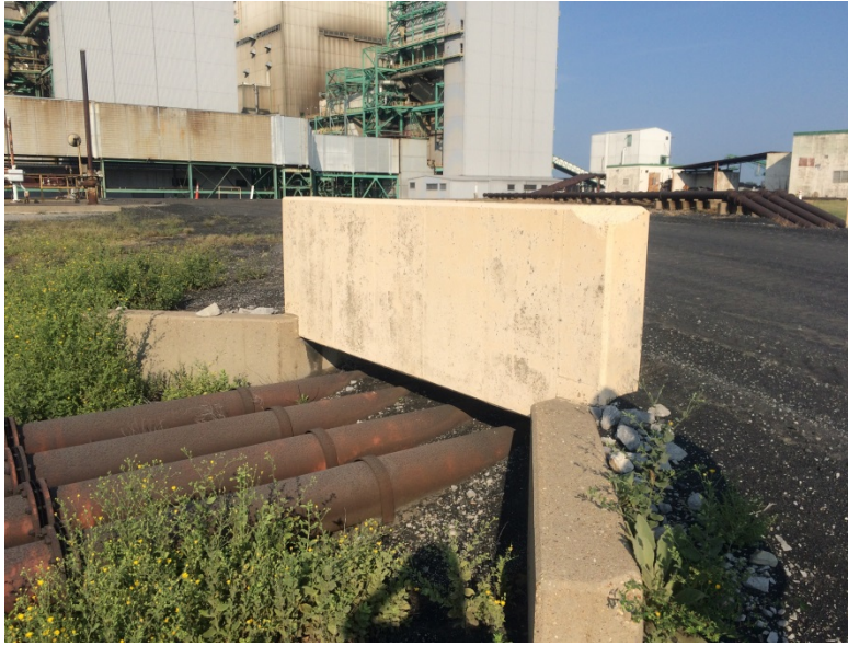
Photograph No. 1 Pond 004 Four inlet pipes with headwall
