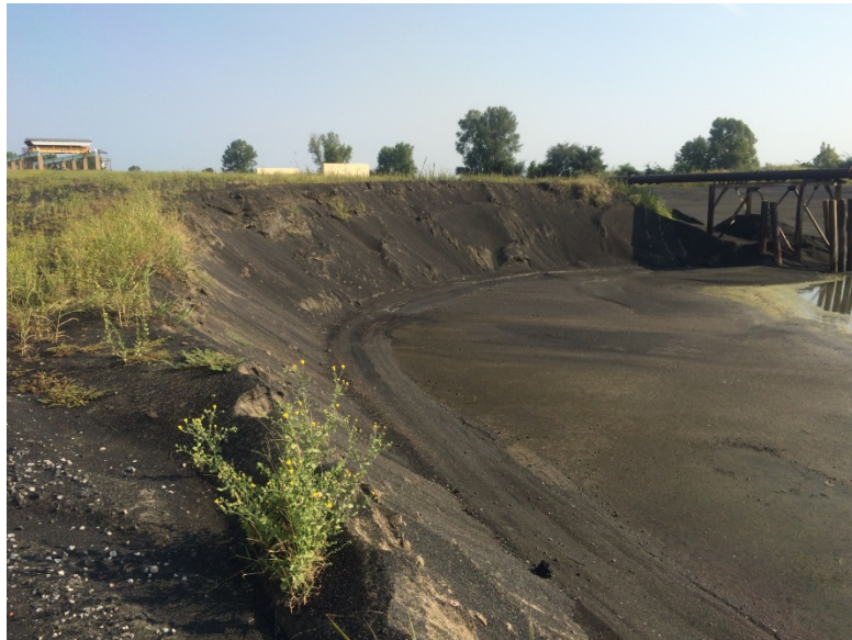
Photograph No. 4 Pond 004 Upstream slope of northern embankment
