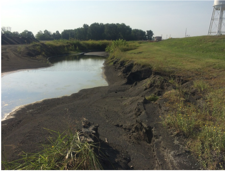
Photograph No. 3 Pond 004 Upstream slope of western embankment
