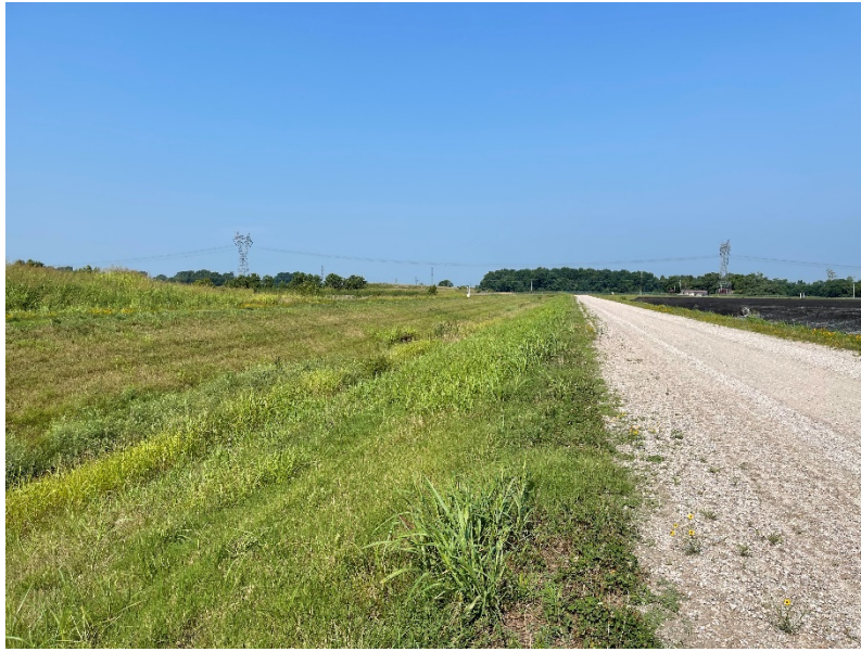
Photograph No. 25 UWL Downstream slope of southern perimeter berm/road of Phase III
