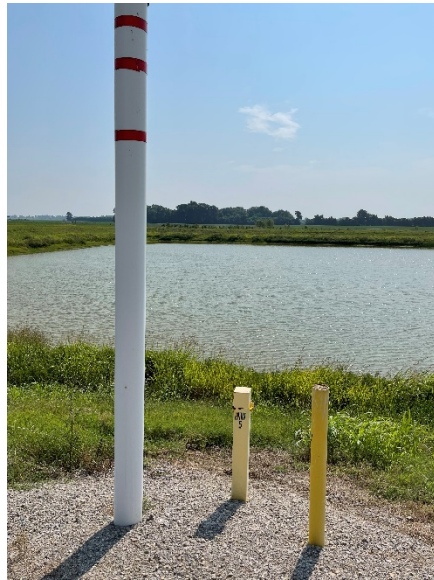
Photograph No. 24 UWL Monitoring well MW-5 Sedimentation pond in background
