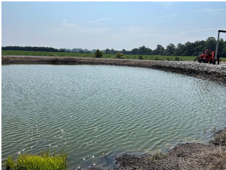
Photograph No. 30 UWL Leachate Pond
