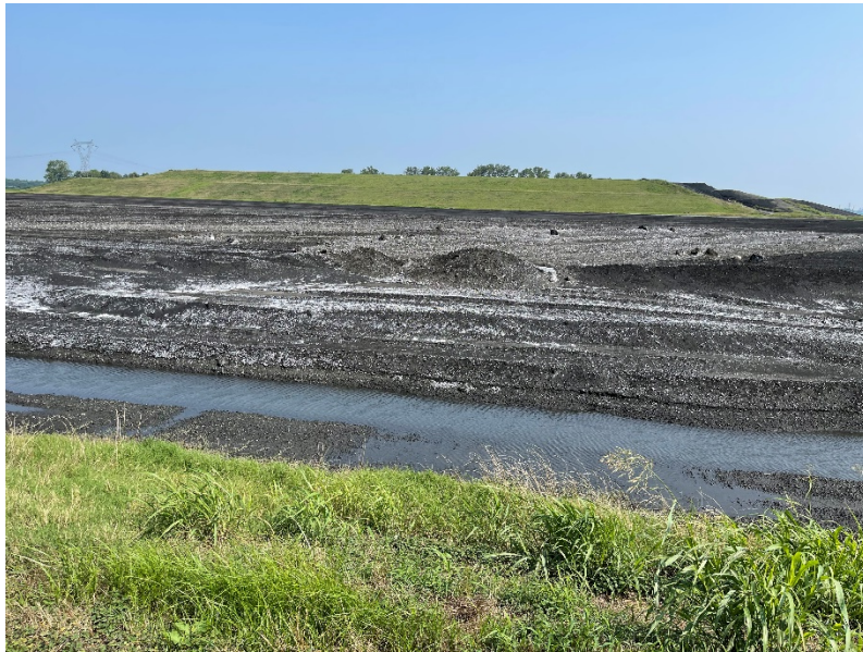
Photograph No. 26 UWL Placement of CCR in open Phase III
