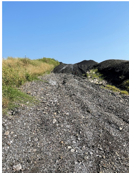
Photograph No. 14 UWL Phase I haul road to top of landfill
