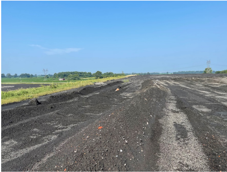
Photograph No. 15 UWL Phase I top of landfill
