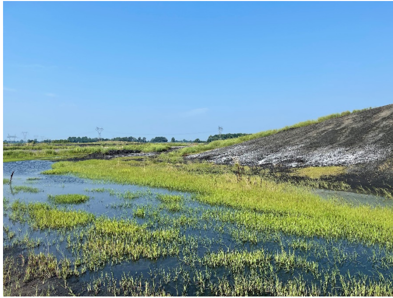
Photograph No. 19 UWL Standing water at southeastern corner of Phase I
