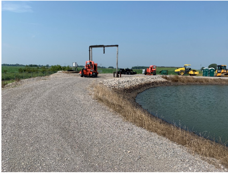
Photograph No. 31 UWL Leachate Pond perimeter berm and loadout structure
