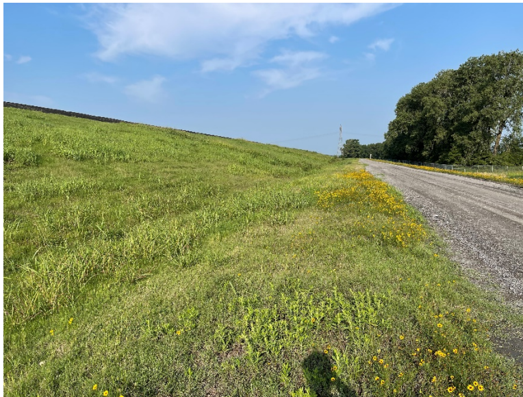
Photograph No. 2 UWL Phase I northern landfill face and perimeter berm/road
