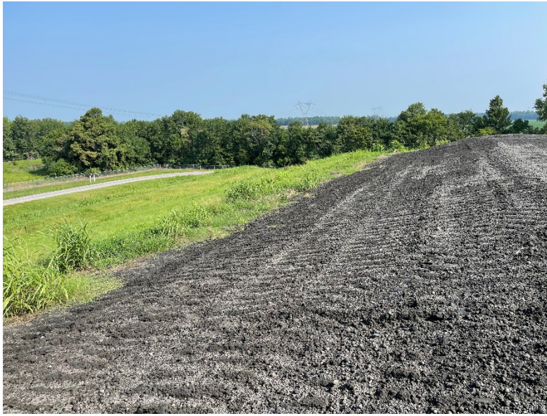
Photograph No. 17 UWL Exposed CCR at top of western face of Phase I
